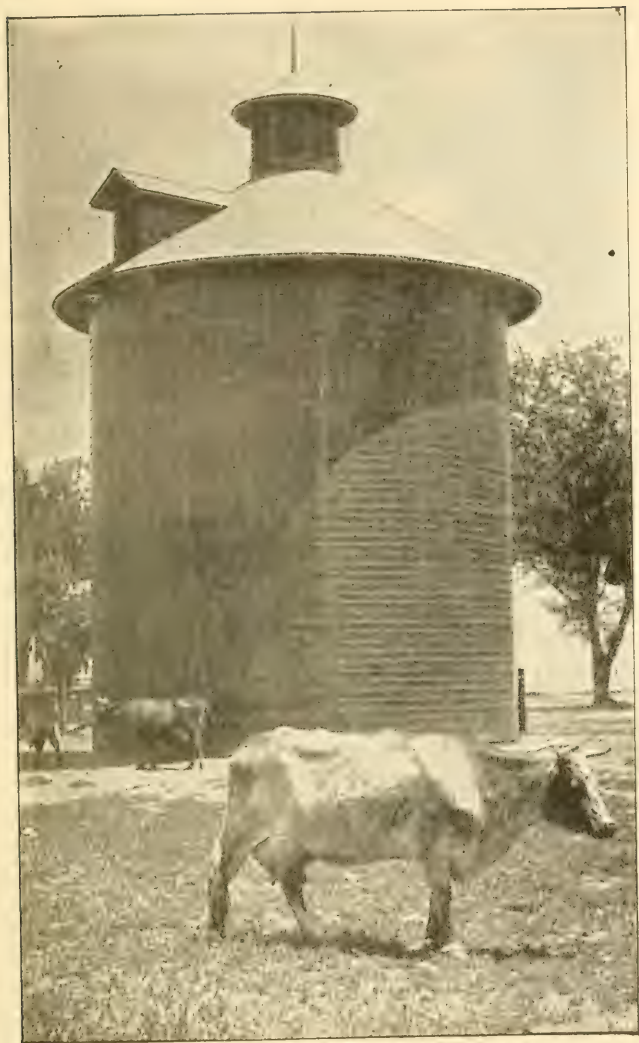
Fig 50—A California Silo Made with Studding
